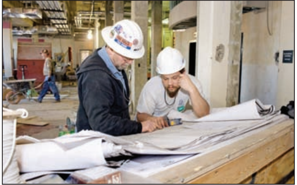
CHECK THE PLANS —Construction workers James Mohler and Pete Cornett look over plans in the front lobby of Cummings Hall, which is closed for a renovation project that includes installing new energy-efficient windows, upgrading bathroom fixtures and providing new mechanical, electrical and plumbing infrastructure.
